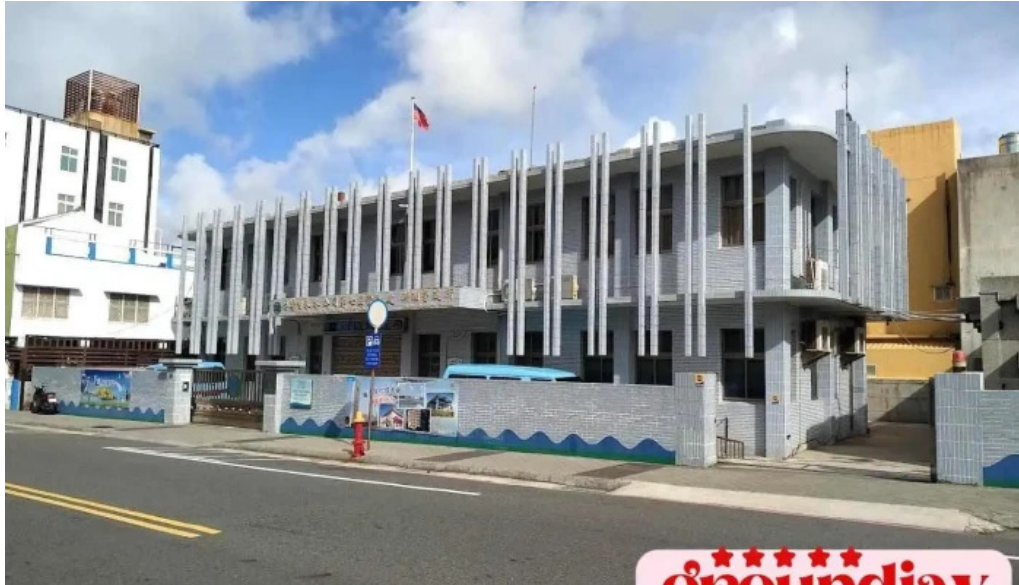
Taiwan water corporation penghu county magong city
