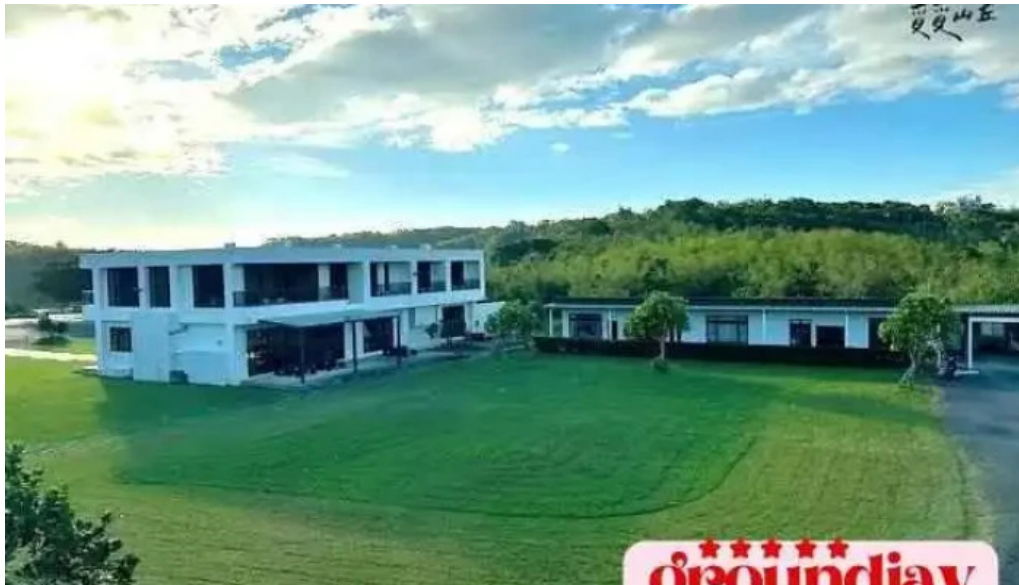
???? ?? ?? still hills inn pingtung county hengchun township
