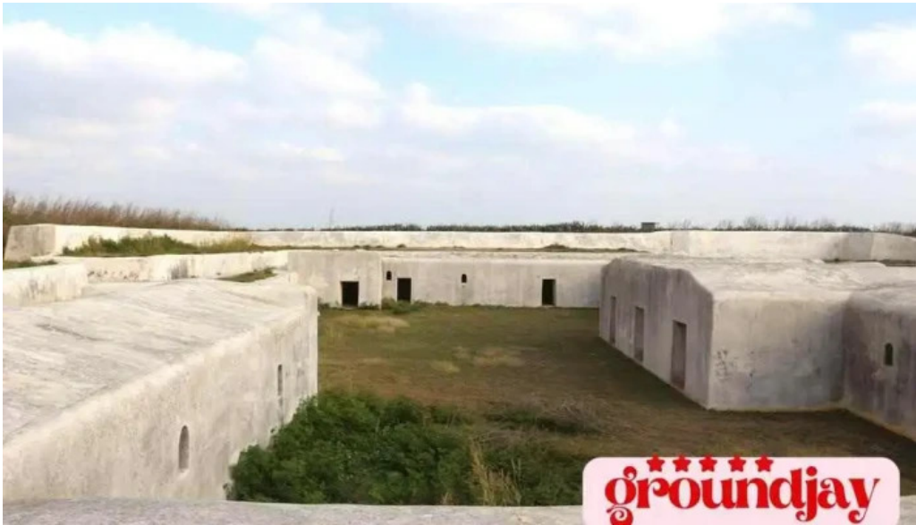
Xiyu east fort ???? penghu county xiyu township
