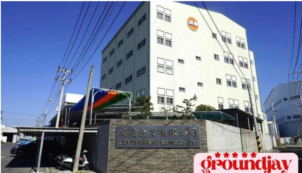
Cetenary electric tainan city annan district
