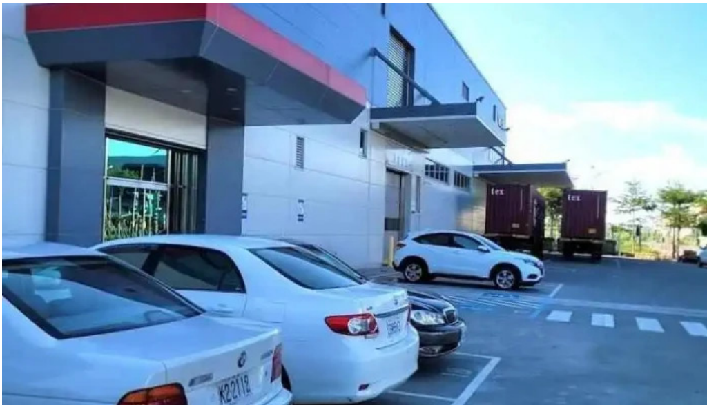
???????????????? kaohsiung city daliao district
